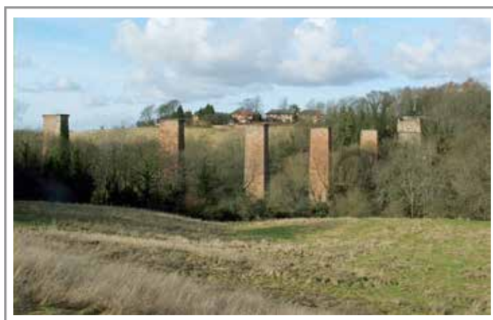
The bridge piers in 2005 before demolition, with Grieve Croft houses behind. The actual bridge was dismantled about the late 60s or early 60s.
